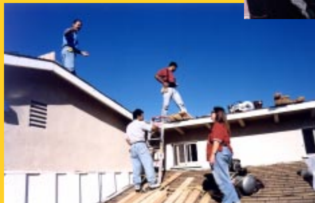
Neighborhood home undergoing soundproofing
